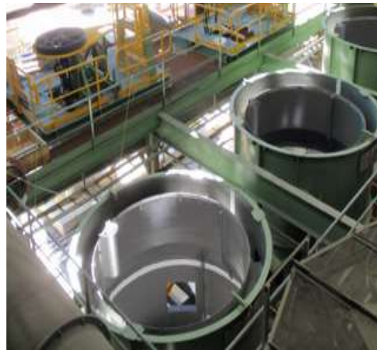
Outotec TankCells during installation
