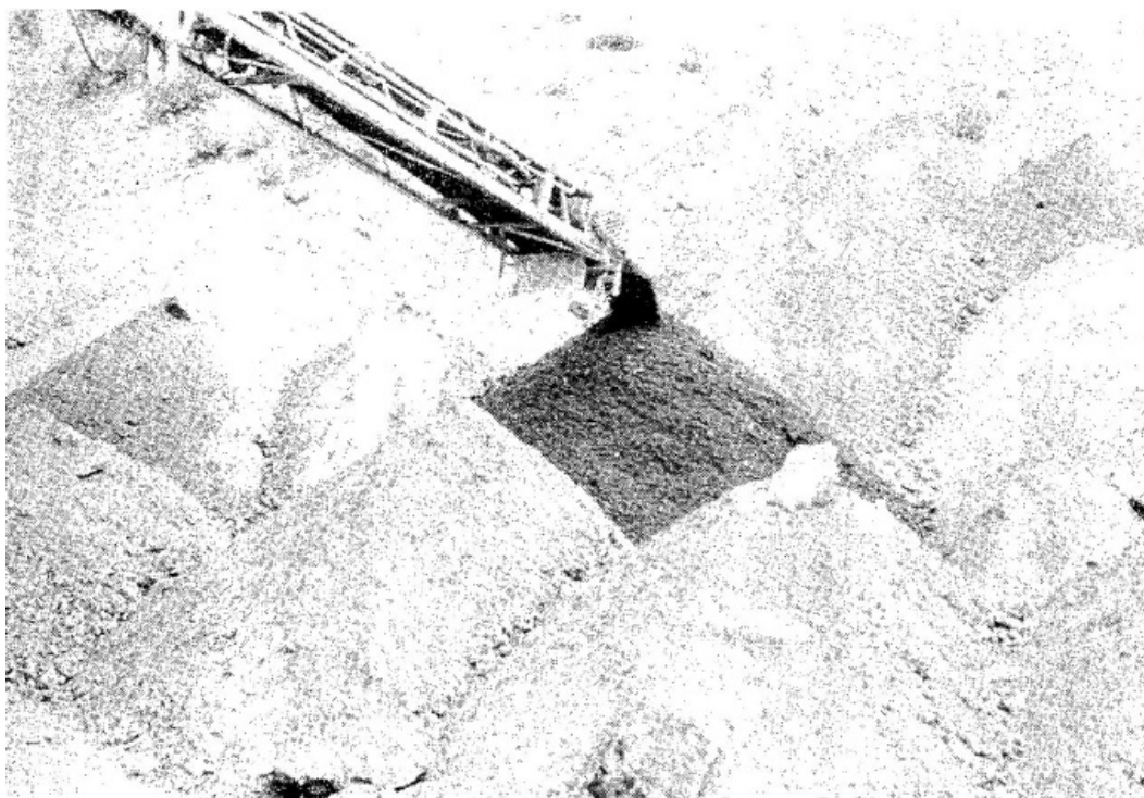
Figure 3. Manual conveyor stacker capable of placing eight tons per hour of mine-run rock.
