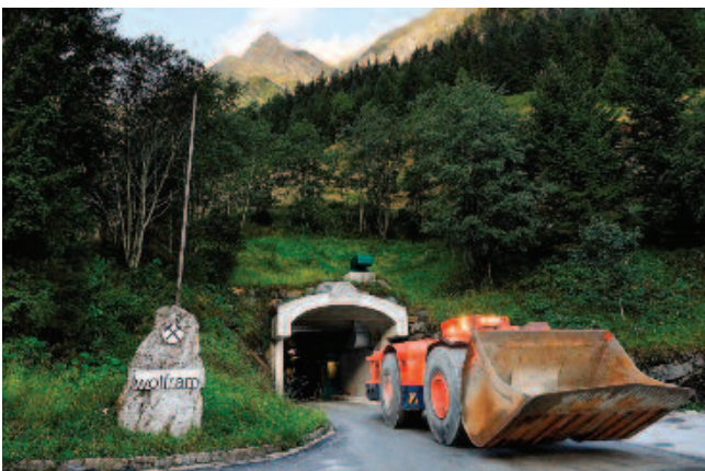
Figure 13: Mine Portal: Mittersill mine, Austria. Access of personnel and material through ramps; ore transport to surface in this case by conveyor belt through a 3km-long tunnel directly to the mill.
