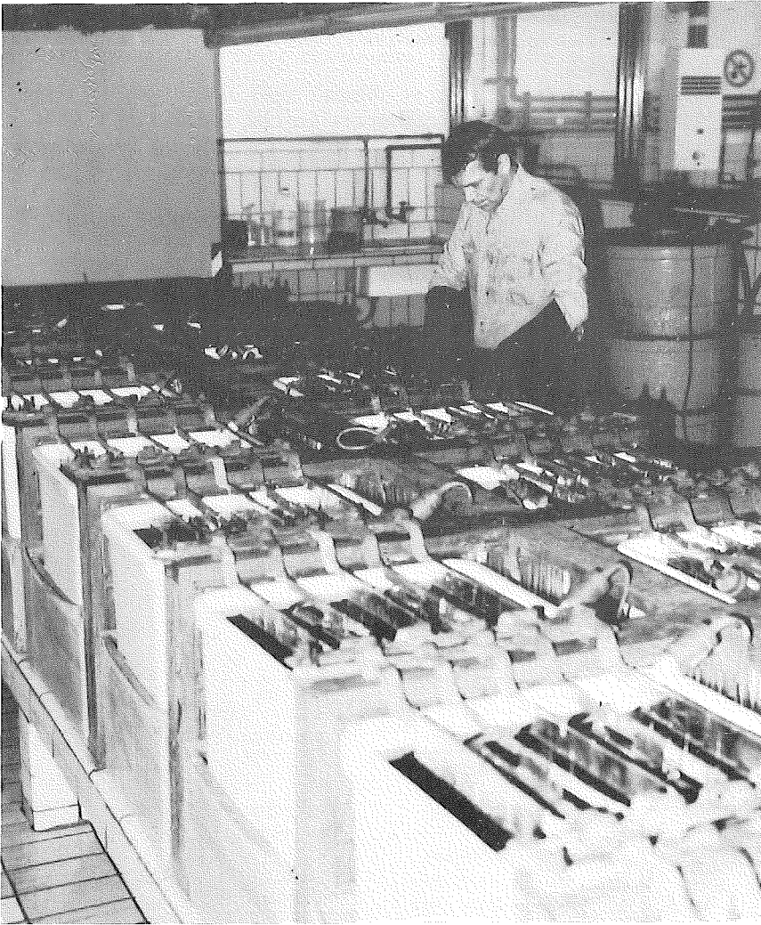
Figure 10.10. Electrolytic gold refining plant.
