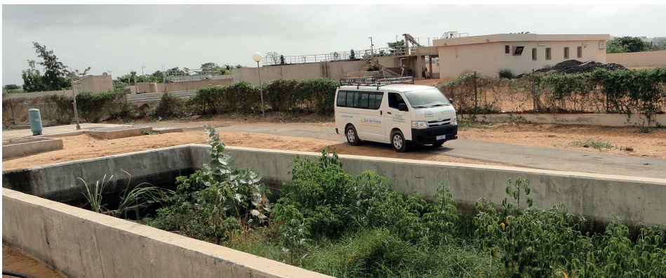
Figure 6.5 Example of inadequate operation and maintenance of a settling-thickening tank in West Africa. The scum was not removed during a long period, which allowed plants to grow on it. The volume of sludge and scum accumulated does not allow for proper operation of the tank, or for solids-liquid separation (photo: SANDEC).
