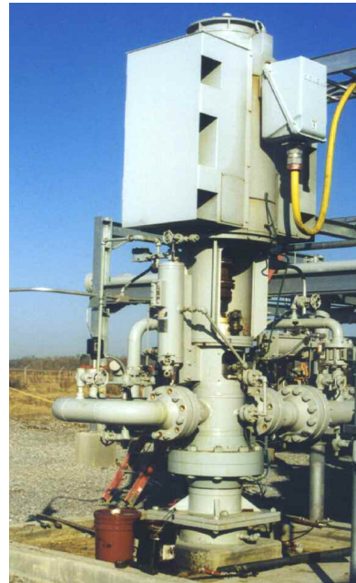
Figure 4. Installation at Pipeline Pump Station.
