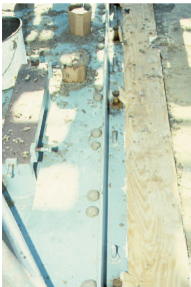
Figure 26. Maintaining Grout Level.
