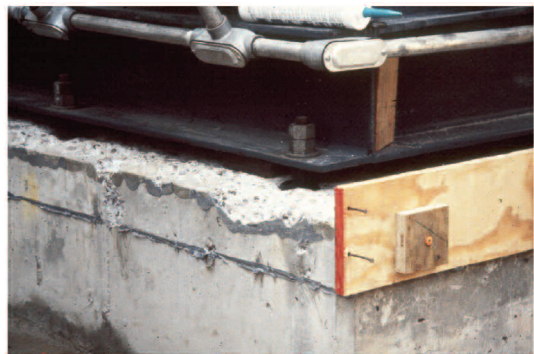
Figure 18. Form Design for a Two-Pour Method.
