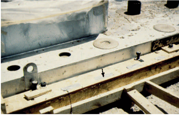
Figure 24. Progression of the Grout in Grout Pour Holes.
