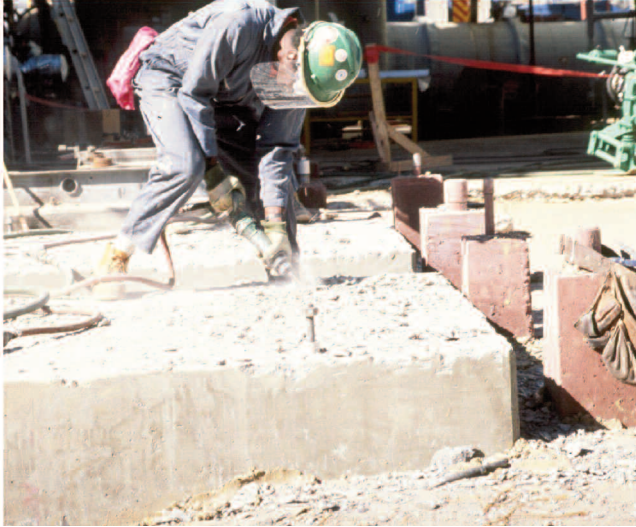
Figure 5. Exposing Aggregate.
