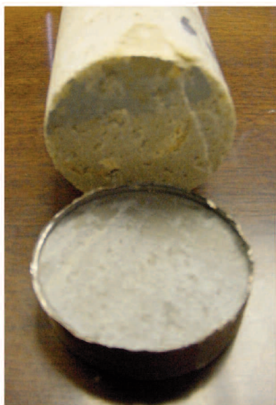
Figure 14. Core Sample Showing Primer Delamination.
