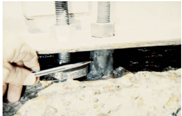
Figure 7. Wrapped Exposed Length of Anchor Bolt.
