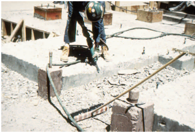
Figure 6. Chamfering of Foundation Edges.
