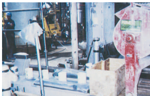
Figure 23. Head Box and Stand Pipes to Produce "Wall" of Grout.
