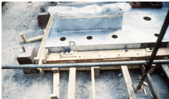
Figure 20. The Top Plate for a One-Pour Grout Form.
