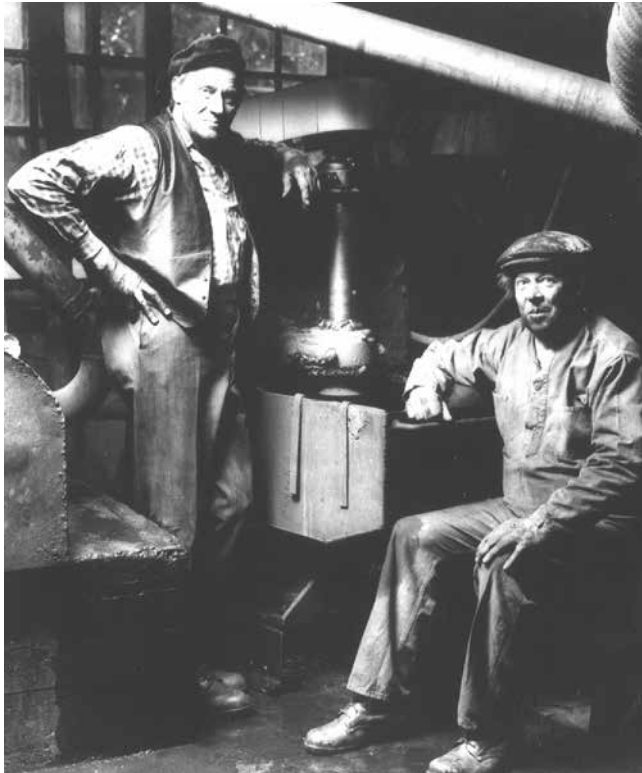
The first vertical pump, manufactured 1933.
