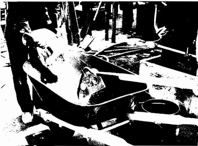
Figure 14. Aggregate Was Slowly Added to the Epoxy and Mixed with a Mortar Hoe.
