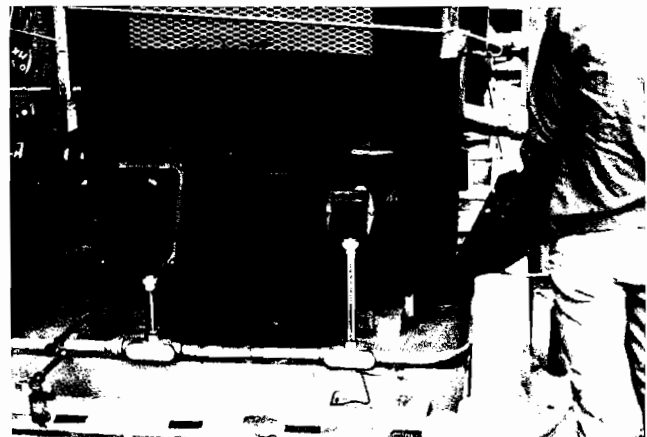
Figure 13. Duct Tape Was Used to Stop Flow of Grout Out Vent Holes as Baseplate Grouting Continued.
