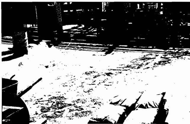
Figure 24. A Sand Path from the Mixer to the Pump Makes Clean Up Much Easier.
