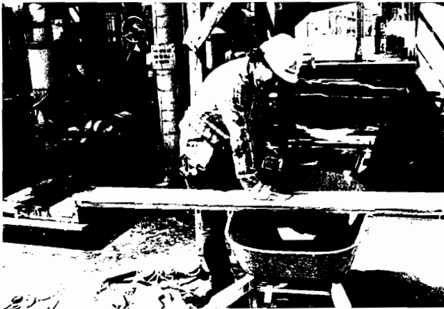
Figure 10. Three Coats of Paste Wax Must Be Applied to All Grout Form Surfaces Coming in Contact with Epoxy Grout.
