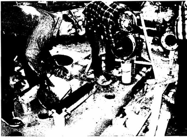
Figure 17. The Resin Containers Are Used to Place Grout in the Center Baseplate Grout Holes.
