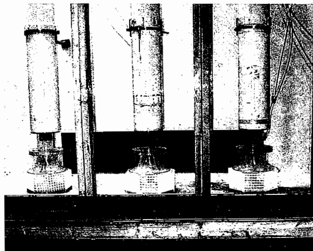
Figure 18. Mod 2 Installed on Pumps.
