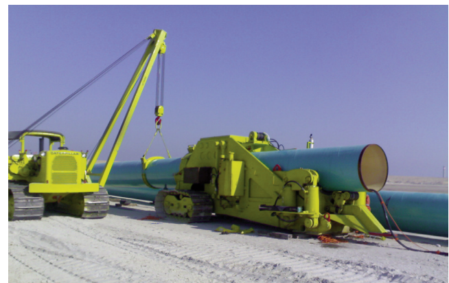
Figure 12. Pipeline Bending Process.
