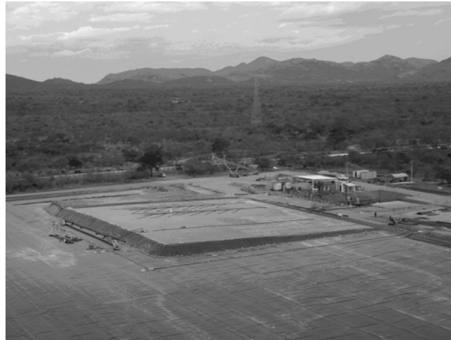
Figure 1: Caraiba Demonstration-Scale GEOCOAT ® Biooxidation Plant (Under construction – September 2008)
