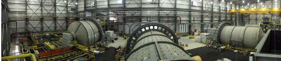
Figure 1 - Overview grinding circuit
