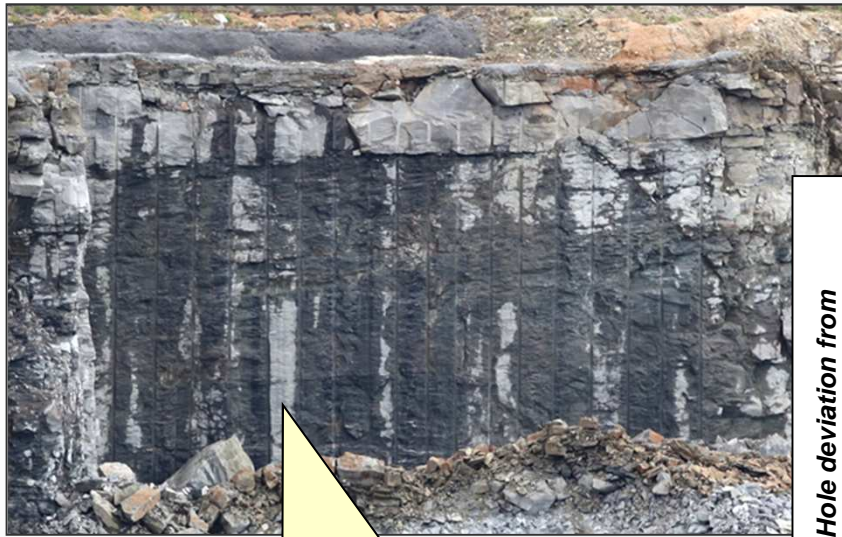
DP1500 - Ø87mm Tubes - 24.5m Bench - Ø140mm Presplit
