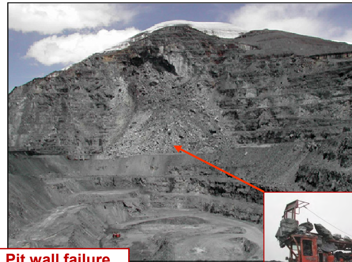
Pit wall failure burying 3 drill rigs in rubble
