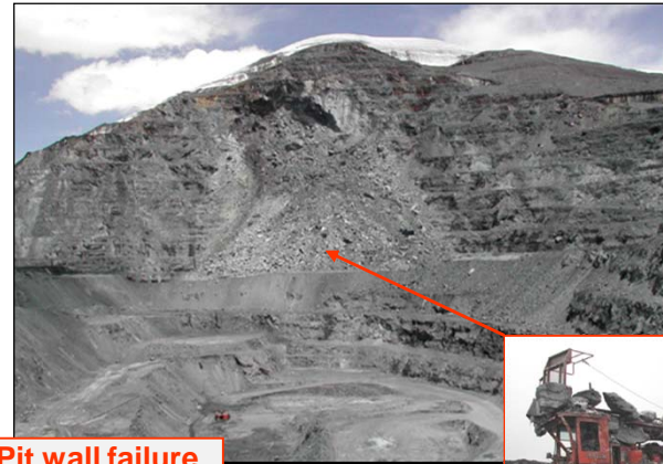
Pit wall failure burying 3 drill rigs in rubble
