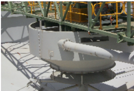
Feed Well & Distributor Cone
